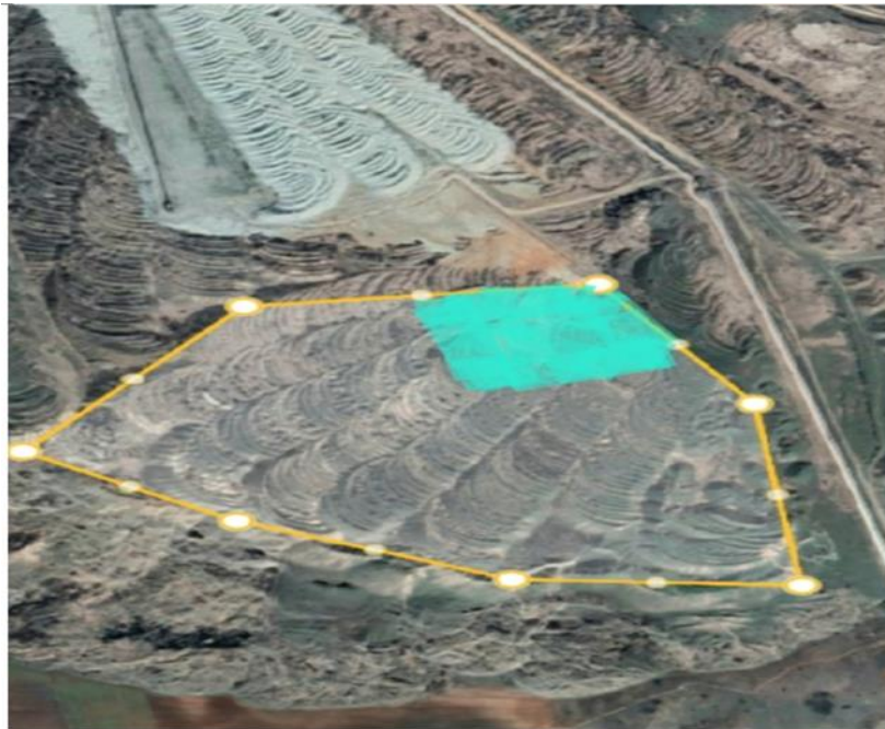
Figure 1. View of the planned location within REK Bitola Compound
