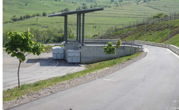
Figure 29 Principle design of a ramp type transfer station
