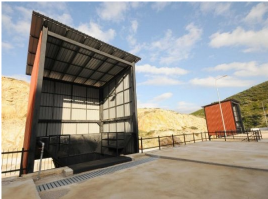
Figure 30 Partly closed unloading area with hopper
