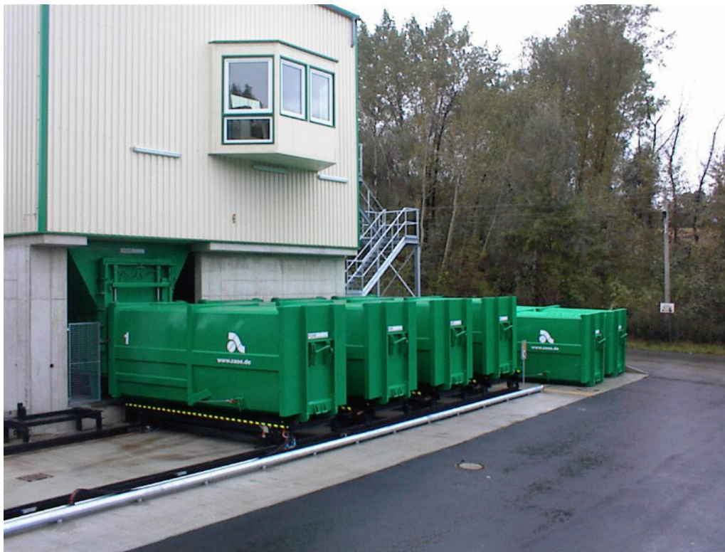
Figure 15 Fully enclosed transfer station with a shifting plant
