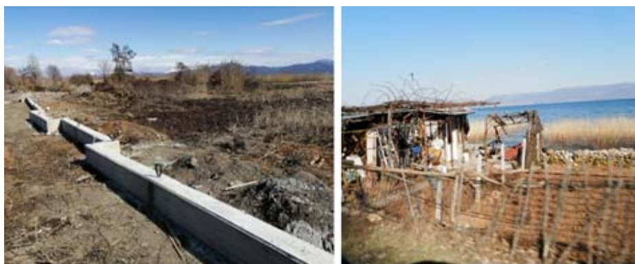
Picture 26. Concrete wall of belt Struga Kaliste and prefabricated house Radožda
