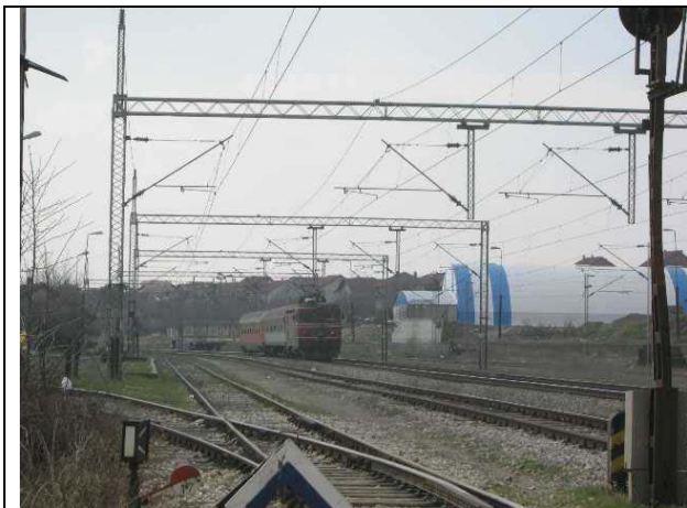
Photograph S1-1. Existing railroad track in the area of Kumanovo
