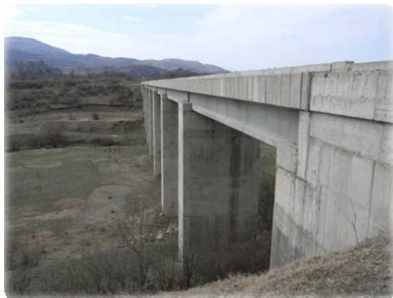
Photograph S2-1. Almost completely constructed bridge over Valley of Kriva river near Beljakovce
