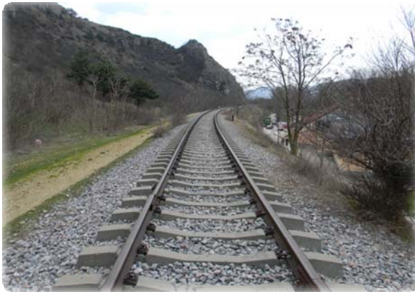
Photograph S1-3. Railroad track above river Kumanovska river in Kumanovo Spa
