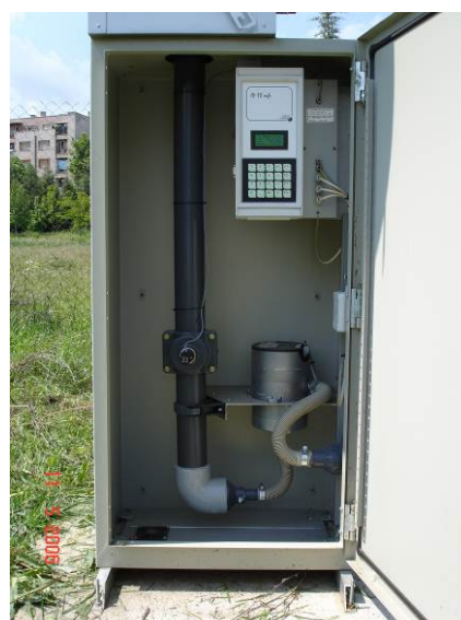
Figure 5-36 Automatic monitoring station in Kumanovo
