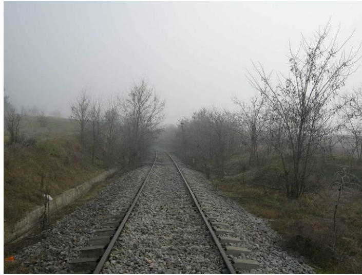
Figure 3-5 Railway Line Rehabilitated Near Kumanovo
