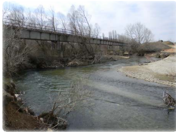
Photograph S1-6. Existing railroad bridge over river Pcinja
