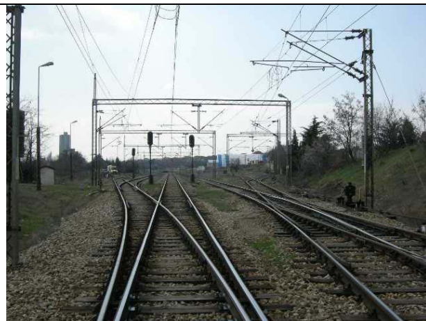
Photograph S1-2. Existing railroad track in the area of Kumanovo
