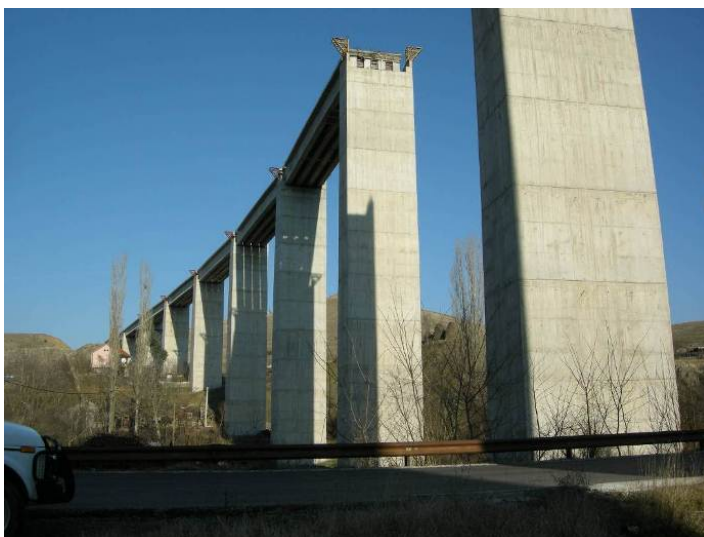
Figure 3-8 Unfinished Bridge near Kratovo Station
