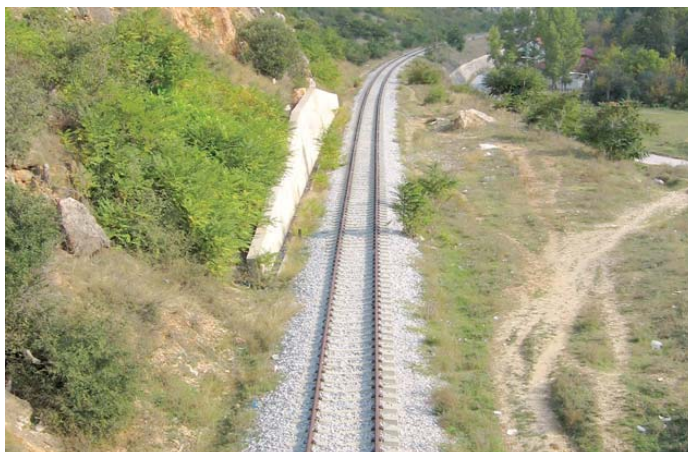
Figure 11-5 Part of Rehabilitated Section Kumanovo - Beljakovce
